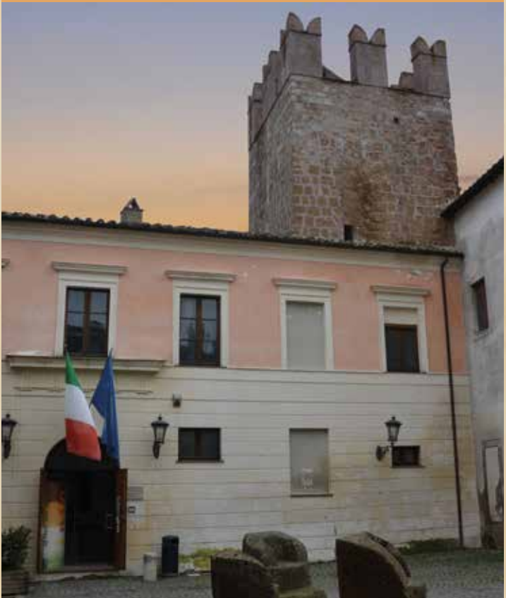
Palazzo Baronale of the Anguillara family in Calcata, seat of the Park offices
