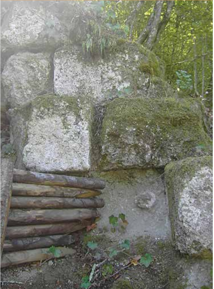
Remains of the Faliscan viaduct on Monte Li Santi hill slope
